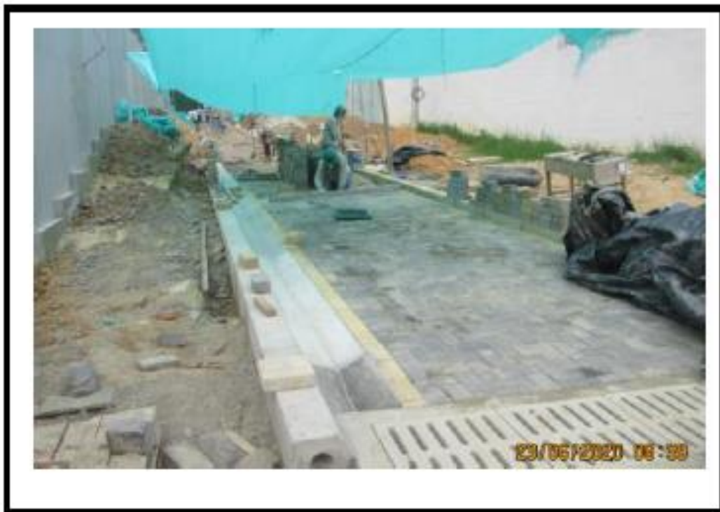
INSTALACION ADOQUINES ANGELES CUSTODIOS
